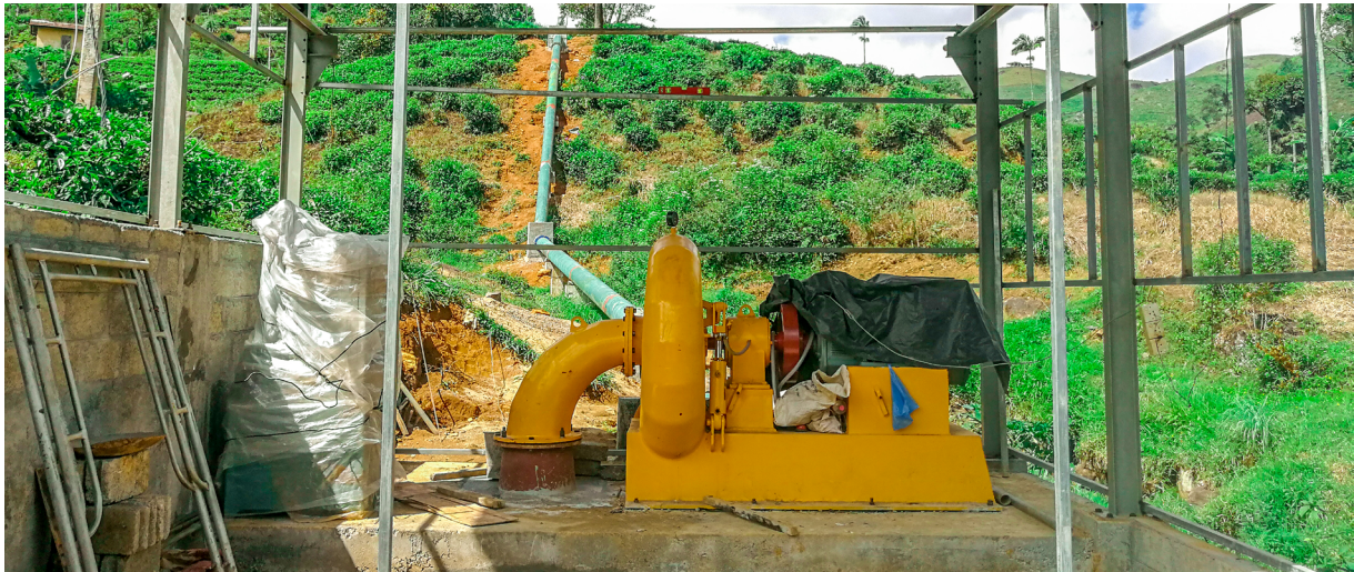
Hydro power plant at Queensberry estate of Kahawatte Plantations.
